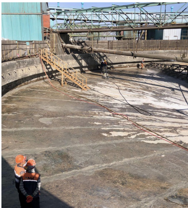
The final preparation step included an aggressive water-jet blasting of the entire surface.
