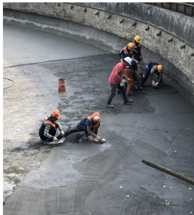
A scrub coat of Megamix II was carefully hand-applied over the entire area.
