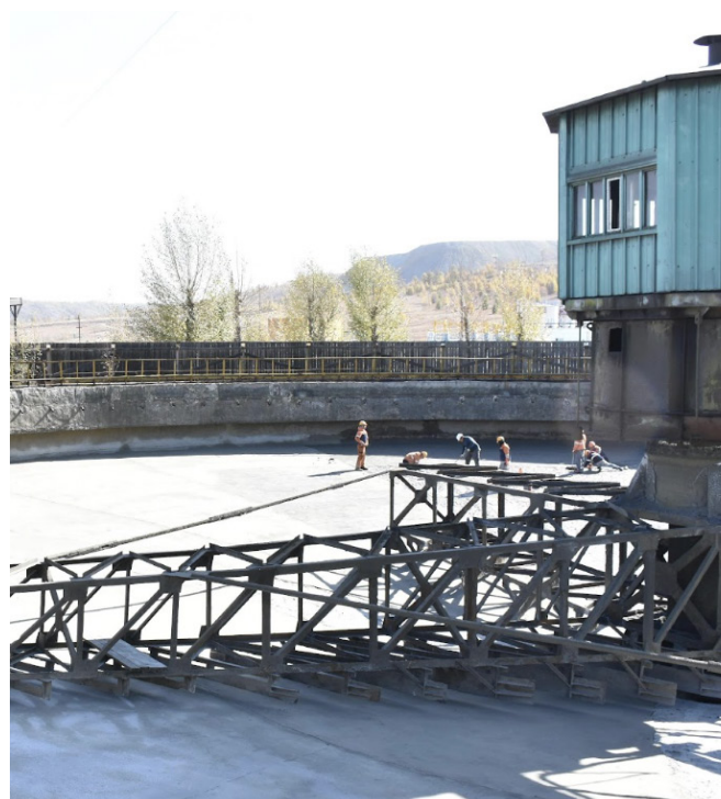
As soon as the Megamix II application had hardened enough to allow for foot traffic, a sprayed application of Xypex Concentrate was applied over the top.
