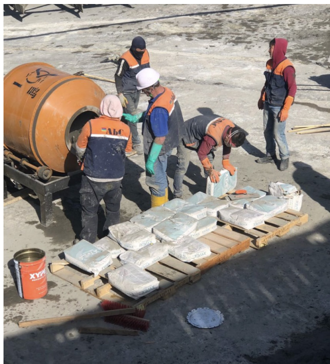
An optimum mix quantity of both Megamix II (6 bags) and water was quickly settled upon and maintained.
